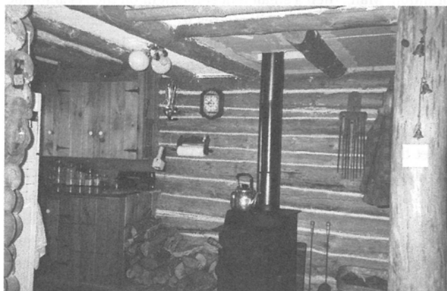
A wood-burning stove helps heat the cabin
