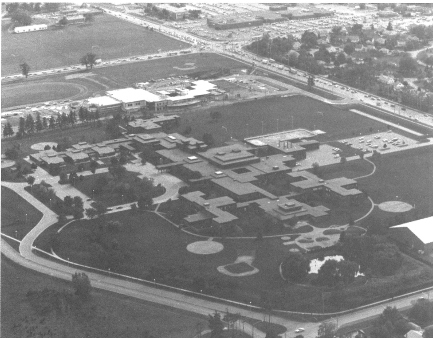
A 1990 aerial view of the Robarts School, London
